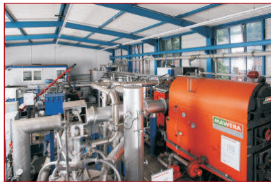
The combustion technology lab at the Institute Branch Sulzbach-Rosenberg of the Fraunhofer Institute for Environmental, Safety, and Energy Technology UMSICHT for examining the combustion and emission behaviour of different biomass fuels ( http://www.umsicht-suro.fraunhofer.de ) ■
