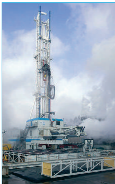
Fig. 1: Drilling rig during testing ■
