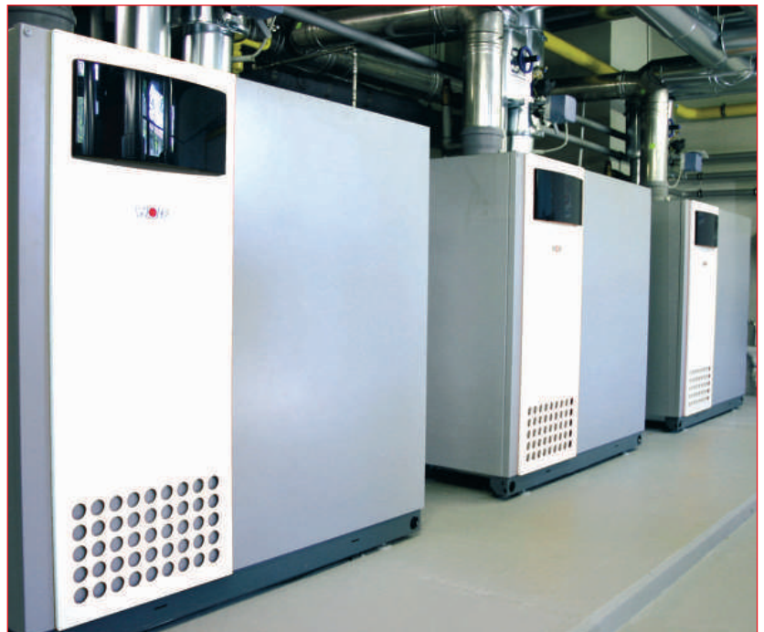
System example: Wolf MGK medium-sized gas condensing boilers in a cascade not only supply plenty of heat but also save a great deal of energy compared to an old heating system ■
