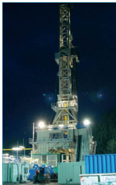
Drilling tower of the geothermal project "Geretsried-Nord" situated south of Munich in order to extract geothermal water for thermal energy and power generation (Gerald Diepolder) ■
