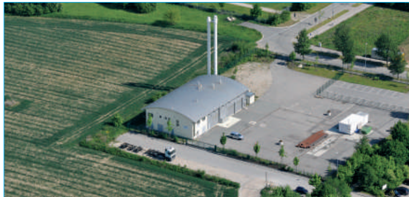
Geothermal heating plant 2 in Erding, Upper Bavaria ■
