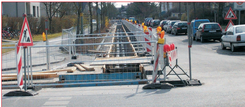
Typical site where a new district heating pipeline is built for the district heating ■
