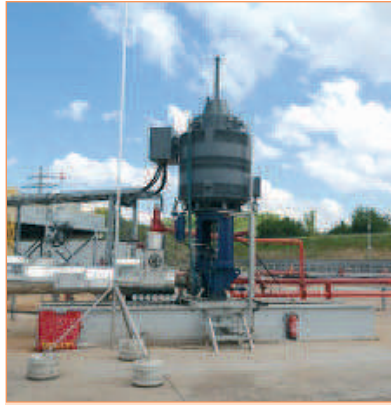
LSP at the geothermal power plant in Insheim with the motor on top of the well. (Source: enerchange) ■
