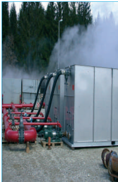
Fig. 2: Cooling towers for the cooling of thermal water ■
