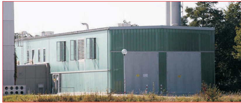
Building for the plant engineering with gas and oil fired boilers as well as heat exchangers ■
