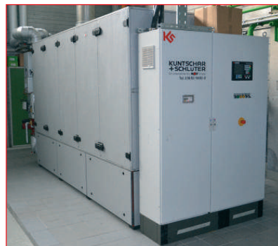
Wolf CHP GTK 240 in situ, with 365 kW thermal output and 236 kW continuous electrical output ■
