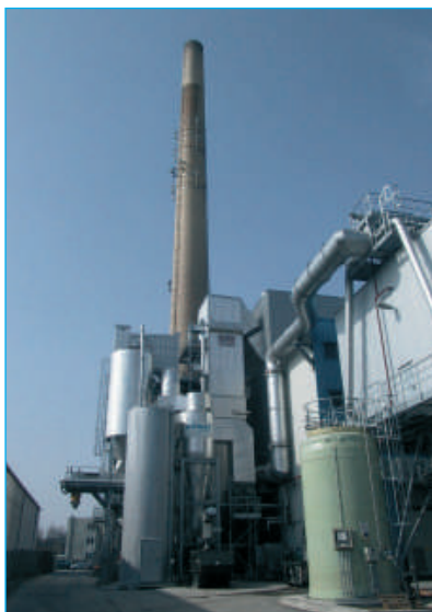
Neufahrn-Eching biomass CHP plant ■
