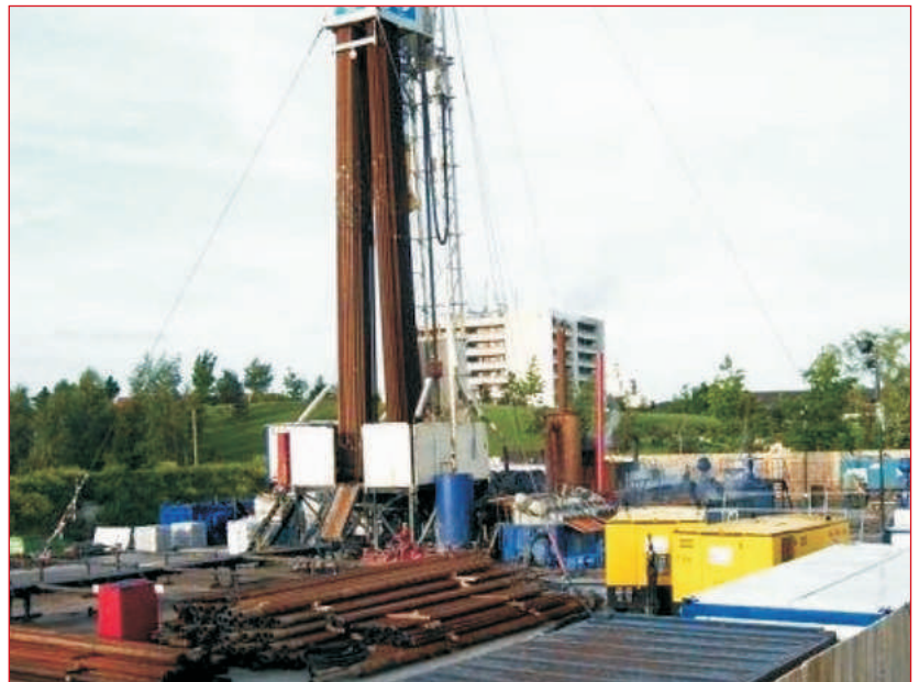
Drilling works for the production well in detail ■
