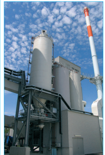
The flue gas treatment system with cooling tower is part of the state-of-the-art RDF power plant. ■
