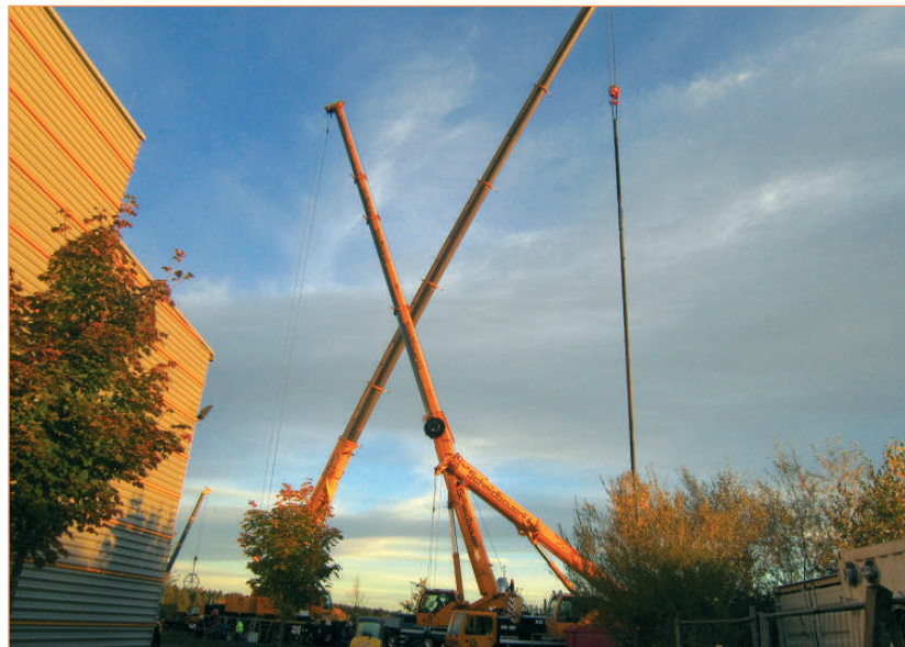
Change of the ESPs at the geothermal power plant in Unterhaching. Due to separate pump garage with a new pump the delay time of the pump exchange was reduced significantly. (Source: Geothermie Unterhaching) ■
