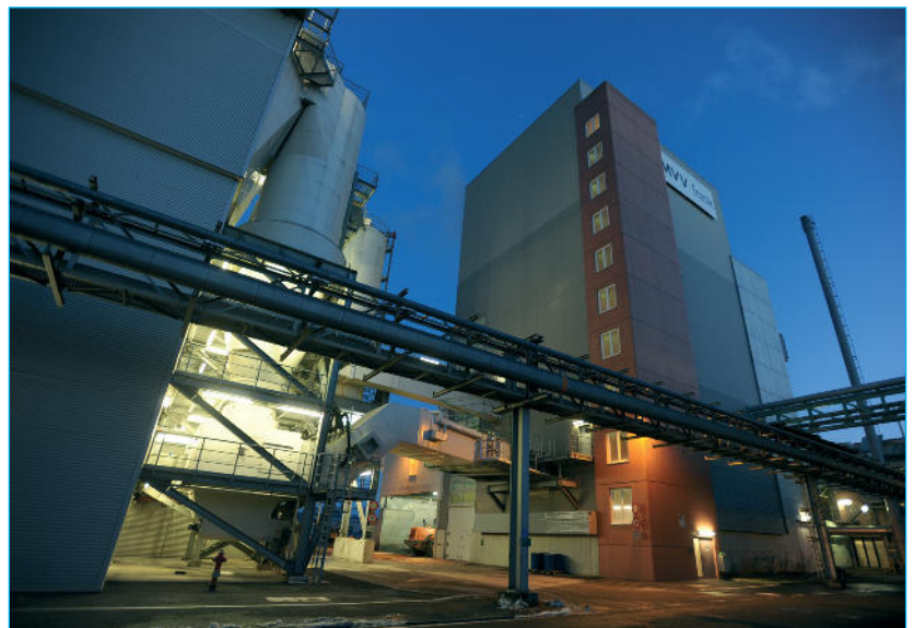
Almost 100,000 tons of replacement fuels can be converted per year to process steam in the MVV Enamic IGS power plant ■
