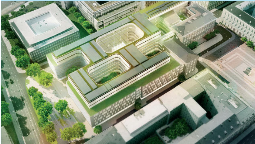
Siemens' new headquarters in Munich will meet highest standards for sustainability ■
