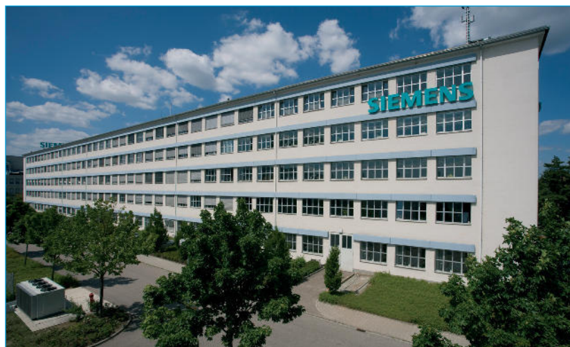
Energy efficiency significantly increased - Siemens' installation equipment factory in Regensburg ■
