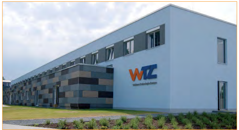
Fig. 1. The building of the Weiden Technology Campus (WTC) ■
