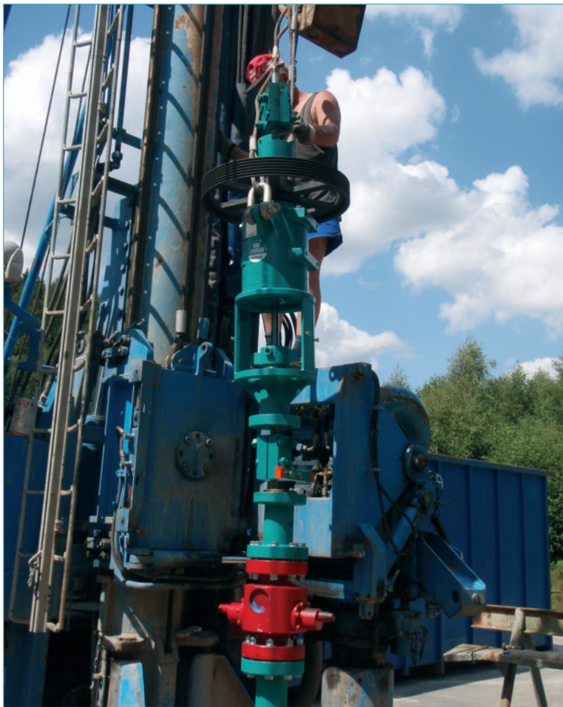
Thanks to the rotor-stator principle, the NEMO® progressing cavity pump is also suitable for the extremely saline, multi-phase medium in the Elster Valley ■
