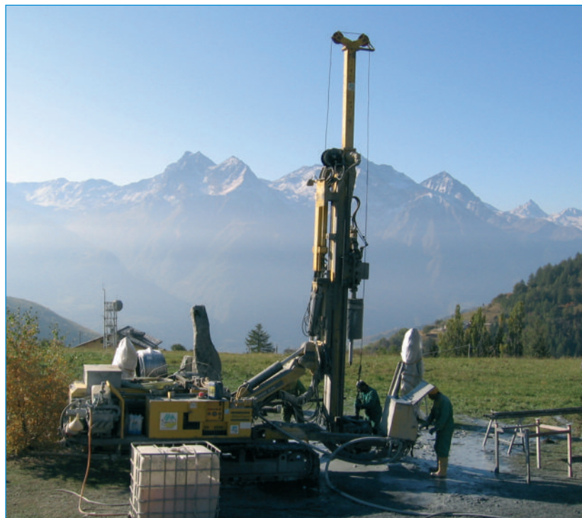
Installation of a borehole heat exchanger in the Aosta Valley, Italy. Copyright: GRETA project. ■
