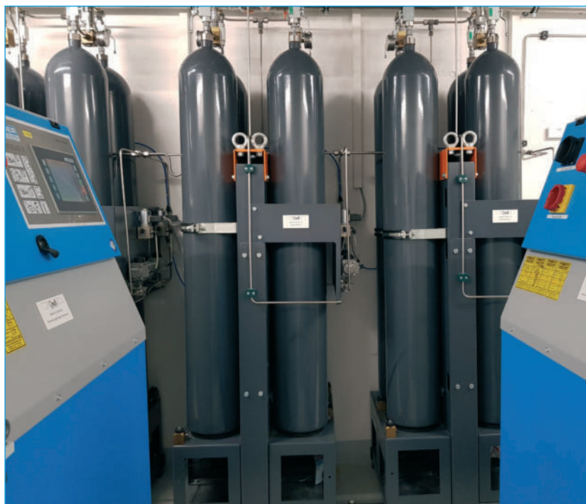
A redundant system of two VERTICUS compressors safeguards production continuity ■
