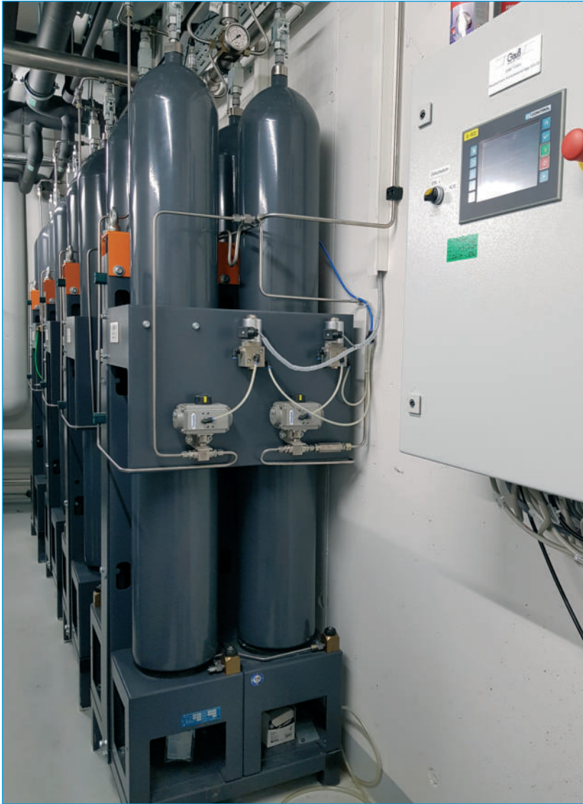
The solenoid valves of the storage rack tanks are controlled by the B-CONTROL unit in fully automated operation. ■
