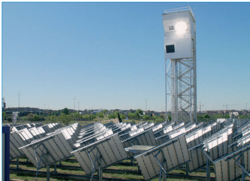
Fig. 1: Research plant for solar-thermochemical jet fuel synthesis (SUN-to-LIQUID research facility, Photo Credit: Christophe Ramage, © ARTTIC 2019) ■
